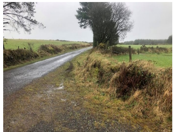
Plate 14-3: Existing Visibility to Right from Proposed Site Entrance at X=3m
